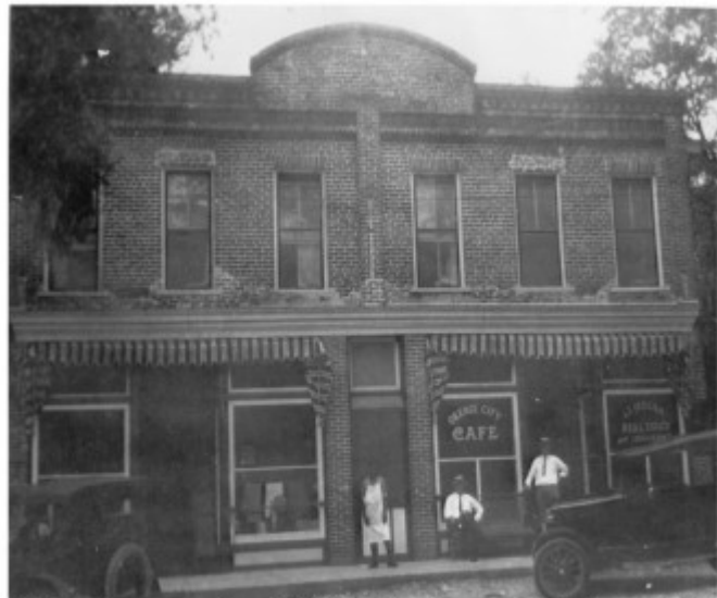
The Clark grocery store building, later known as the Hogan Hotel [From the Orange City Library Association collection used with permission of Mr. Harley Strickland, President and thanks to Mrs. Joan LaFleur]
