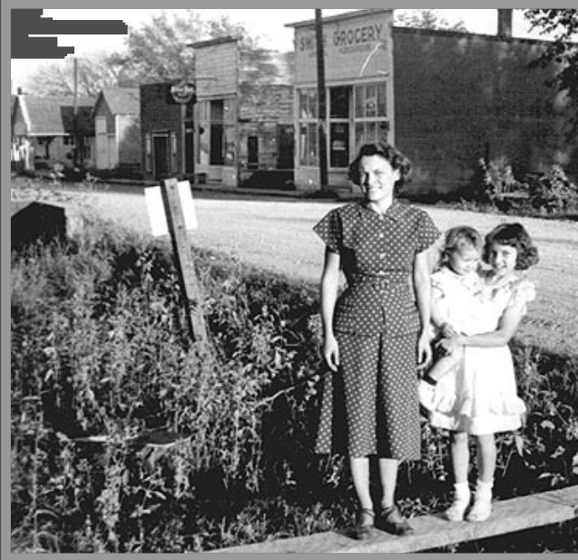
LaVonne, Lois holding Joanne at Colwell, Iowa — the buildings from left to right are the creamery and lockers, trolley tracks (the trolley once ran from Colwell to Charles City), post office, welding shop, 2-story saloon, vacant lot where Wm. Elbert Todd once had his blacksmith shop, the Smith's Grocery. On the other side of the street was the Shell Station, Wondroe's Produce, Kral's Tavern, Kapka's Store, Easterly's Hardware & Tractor and the Elevator
