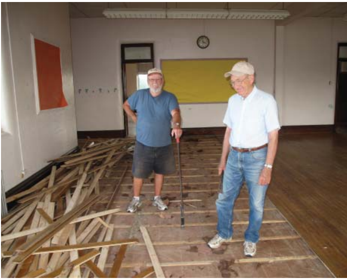
Howard Durham and Maurice Welsh look over the maple floor they removed from Mrs. Harter's 6th Grade room
