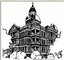
1896- Denton County Courthouse-
