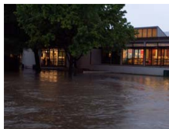
South view of the library
