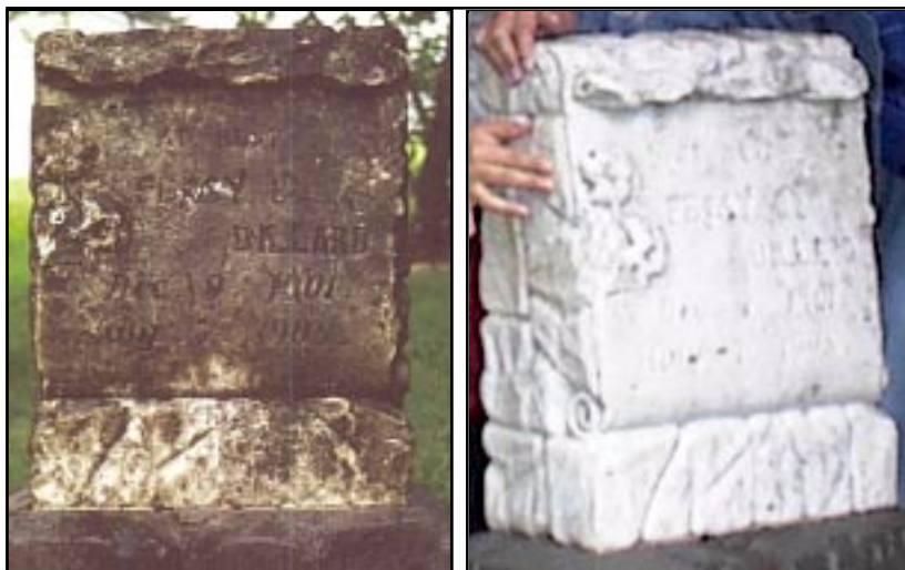
Left: Marble headstone covered in dirt, grime, and black moss. Right: Headstone after cleaning with water, then non-ionic detergent, then household ammonia, and finally to destroy biological growth, with calcium hypochlorite.
